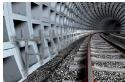
Instalace v tunelech
